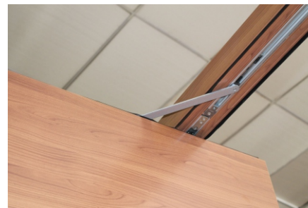
Concealed closing mechanism
