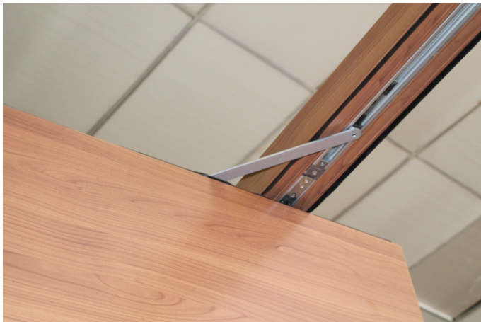
Concealed closing mechanism
